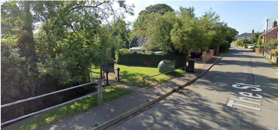
Figure 11 - The Street, Woodton showing run off culvert (left) and looking towards historical flooding zone
