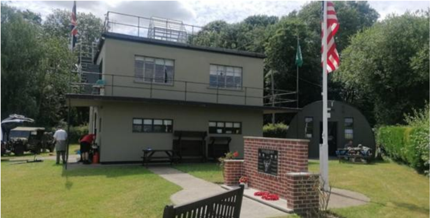
Figure 22 – Seething Control Tower and Memorial Garden
