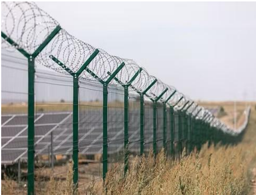
Figure 19 – Typical Solar Farm security fencing
